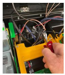
Once confirmed, tighten the cable tie.
